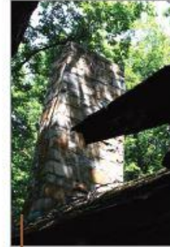
The chimney of the Carriage House, like all fireplaces and chimneys of the Lodge, was made of Vermont stone.
