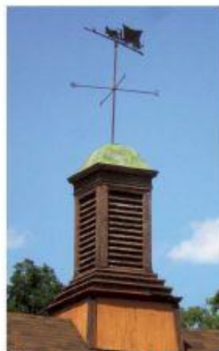
The attractive cupola, still present on the building, provided draft-free ventilation.
