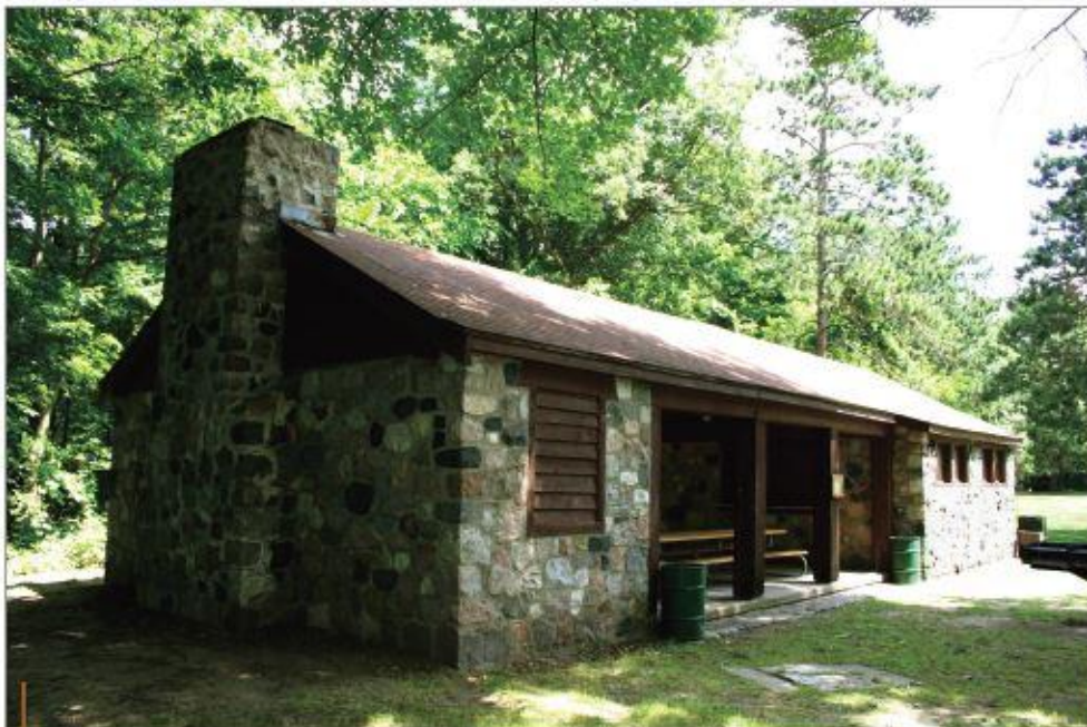
This pavilion was built in the 1930s by the Civilian Conservation Corps. The pavilion has offered shelter, bathrooms, and views of the natural scenery to visitors for generations.
